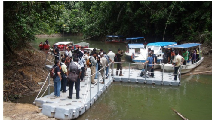
New pontoon jetties provided at Royal Belum State Park to boost visitation (Photo by: Amran Hamzah)
